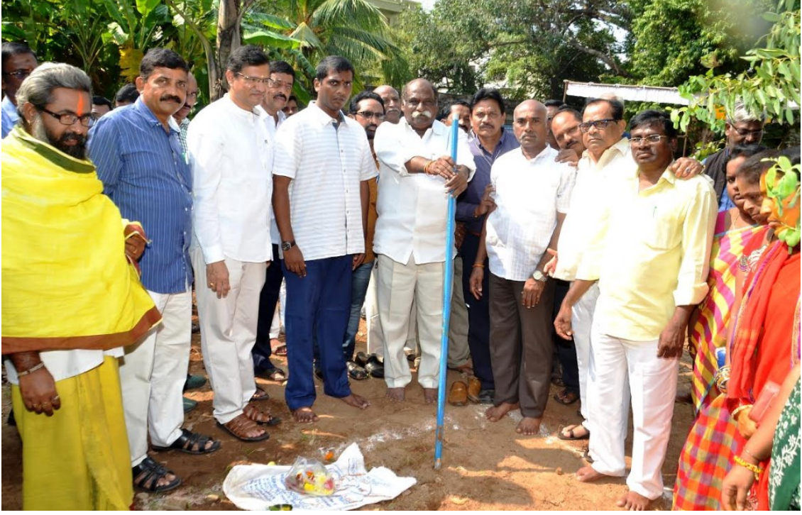
MLA East Velagapudi Ramakrishna Babu Laying Foundation stone to 2600 KL capacity New GLSR at asilmetta Reservoir Along With GVMC Commissioner Sri M Hari Narayanan.
