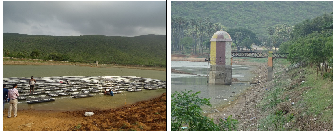
Ongoing construction of 2MW floating solar park on lake
